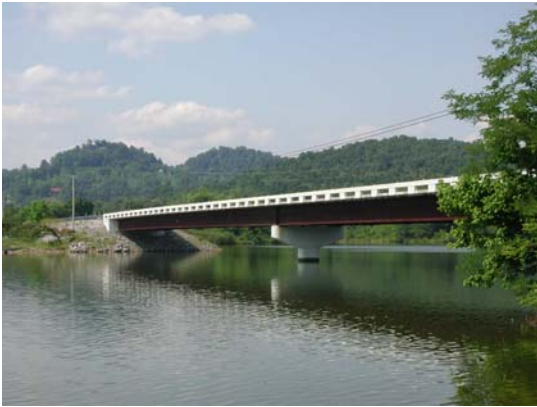
Martins Creek Bridge SR-53
