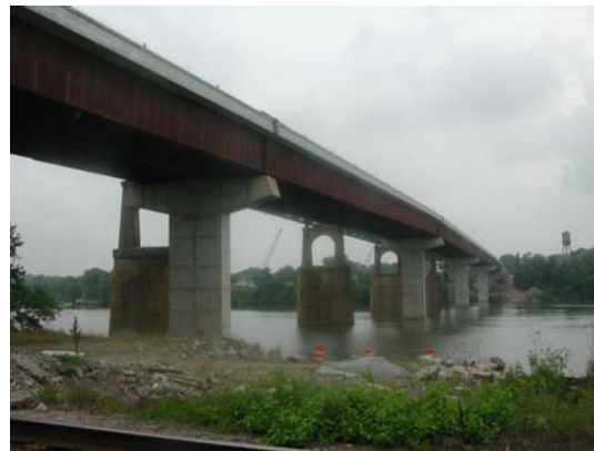
Loudon County Bridge SR-2 over Tennessee River
