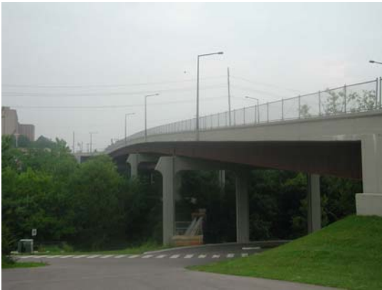
Third Creek Bridge SR-450 Knoxville
