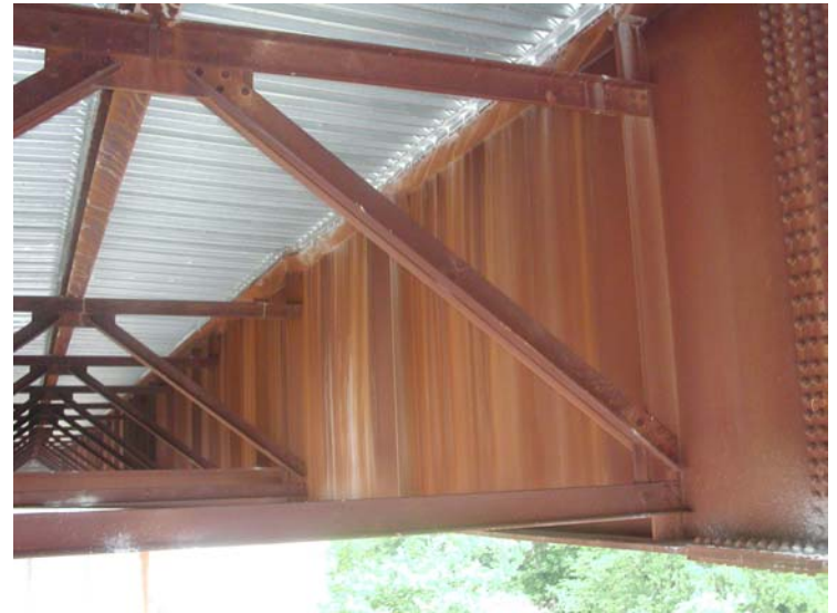
Paint/Leakage
