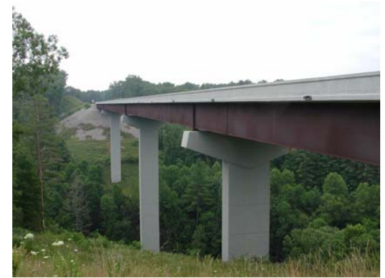
Clear Fork River Bridge SR-52
