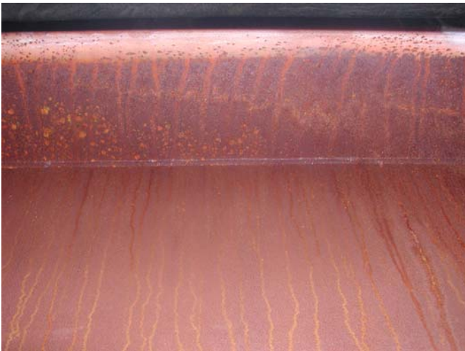
Condensation/leakage
