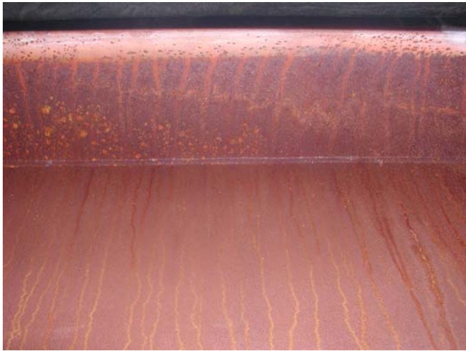
Condensation/leakage
